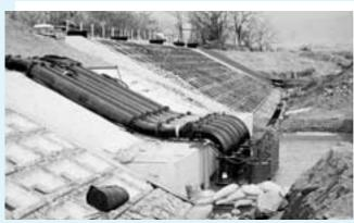
Because of its robust construction, B-series pumps are sometimes used for dewatering in construction site. Compact shape allows high portability comparing against the horizontal pump which requires a firm installation foundation work. In such case, some pump parts are changed its material into harder materials.
