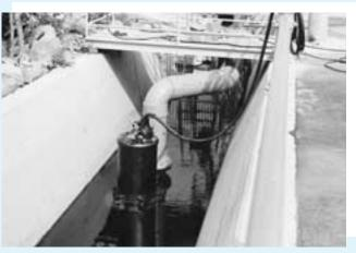
B-series pumps being used for a temporary installation during rainy season.
