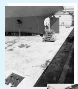
In the shipyard, B-series pumps, which are operated by fully-automatic control, work for level control and dry up. For sea water, sacrificial anodes are applied.
