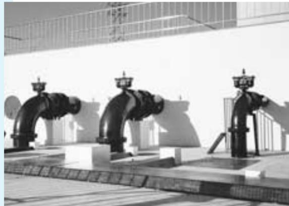
As it is silent during operation owing to its underwater operation, B-series pumps are often used at the basement of buildings in the city area.
