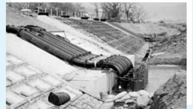
Because of its robust construction, B-series pumps are sometimes used for dewatering in construction site. Compact shape allows high portability comparing against the horizontal pump which requires a firm installation foundation work. In such case, some pump parts are changed its material into harder materials.
